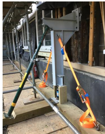
One of the jacks in place during the restoration work
